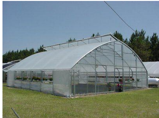
#8 Free-standing Frame Structure
