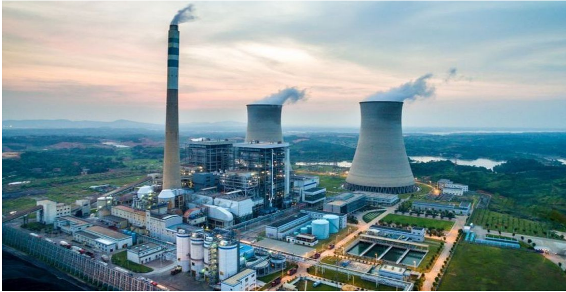
Figure 2 Nuclear Power Plant 14
