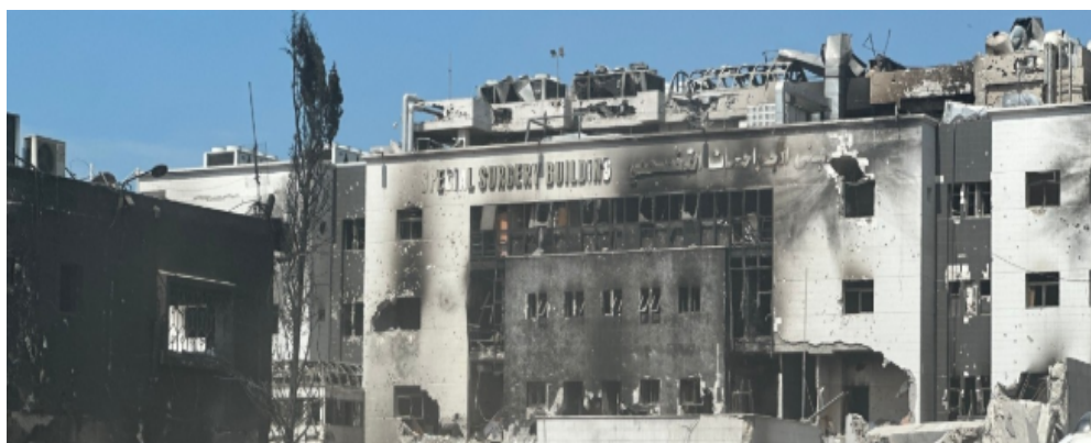
Figure 1 26 : Image depicting a destroyed hospital in Gaza after an aerial attack
